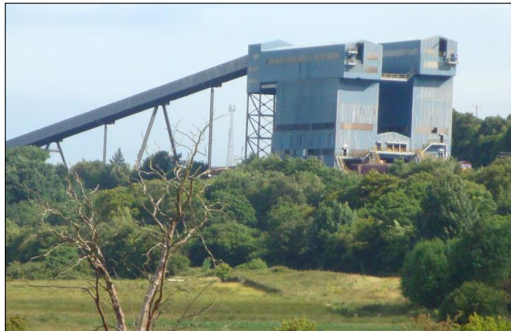
Capable of accommodating five trains simultaneously, the Hunterston rail car loader system includes multiple bunker feed conveyors and provides rapid filling of 100 ton and 44 ton railcars.
